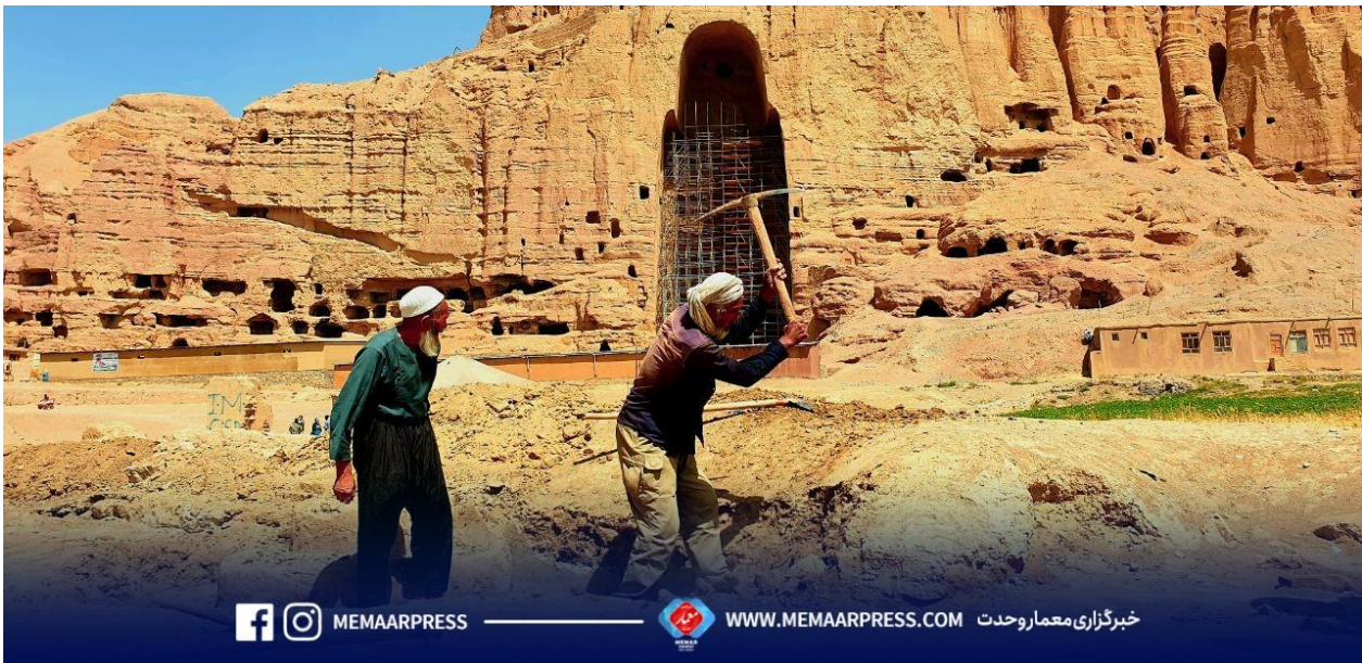
Destruction of the ancient areas around the Bamiyan Buddha after the Taliban ordered to build a market in the protected area (photo by Memaarpress).
